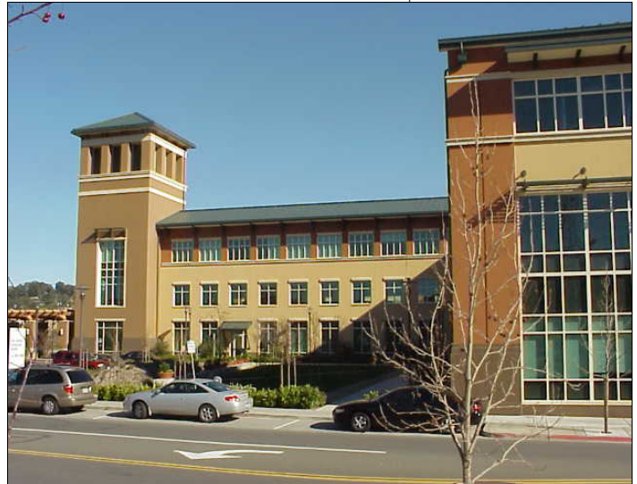
The San Rafael Corporate Center, a Class A office development, is a redevelopment of a Brownfield site in Downtown.
