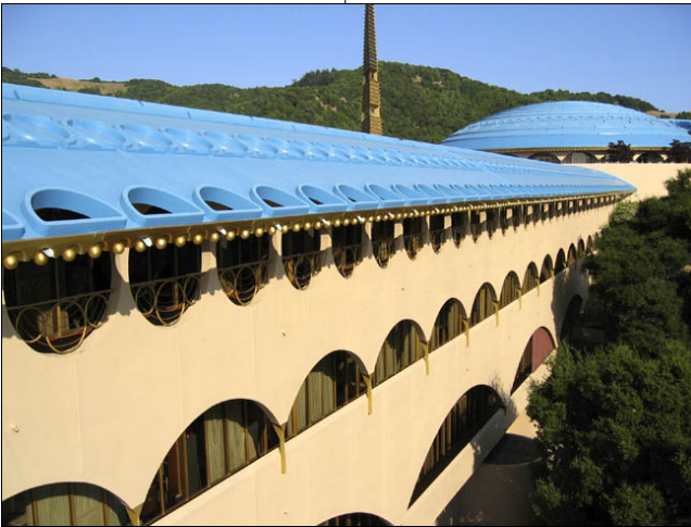
The Marin Civic Center is the only public building designed by Frank Lloyd Wright to be built.
