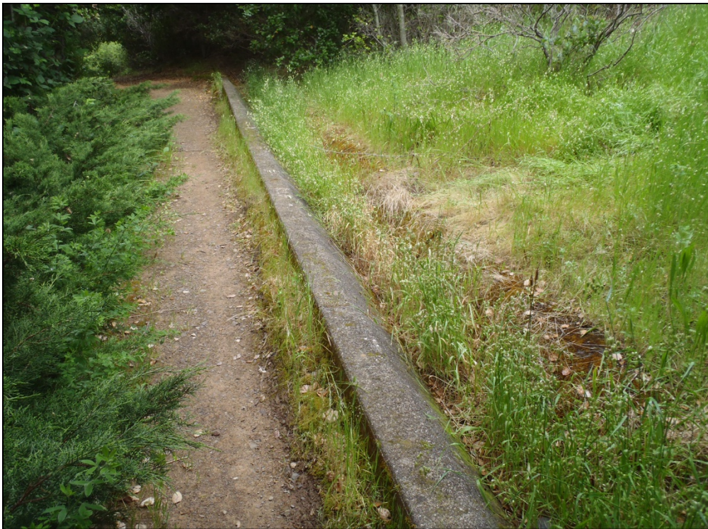
Photo 5. Modern concrete ditch extension east from ditch intersection/angle point, view east
