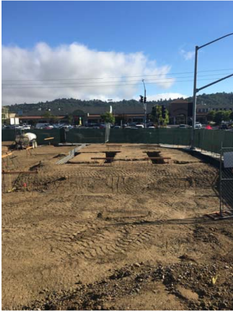
July progress pictures – site work, grading and footing excavation at FS 52
