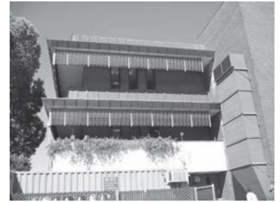
East entrance from police parking area.
