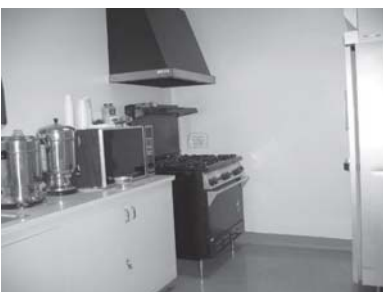
Kitchen is inadequate for shelter needs
