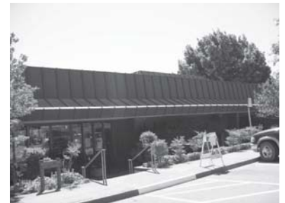
Difficult wheelchair access from parking lot.
