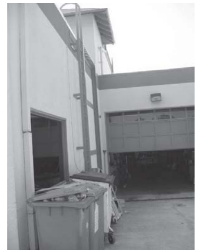
The service/mechanic's areas are extremely small; this operation will move to Fire Station No. 2 by 2022.
