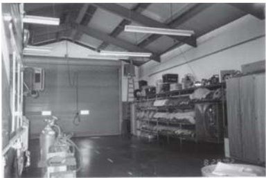
Hose storage in apparatus bay
