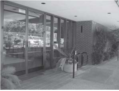
North public entrance
