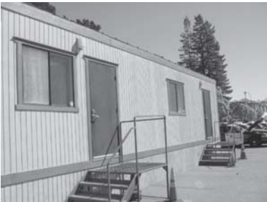
Modular unit in parking lot
