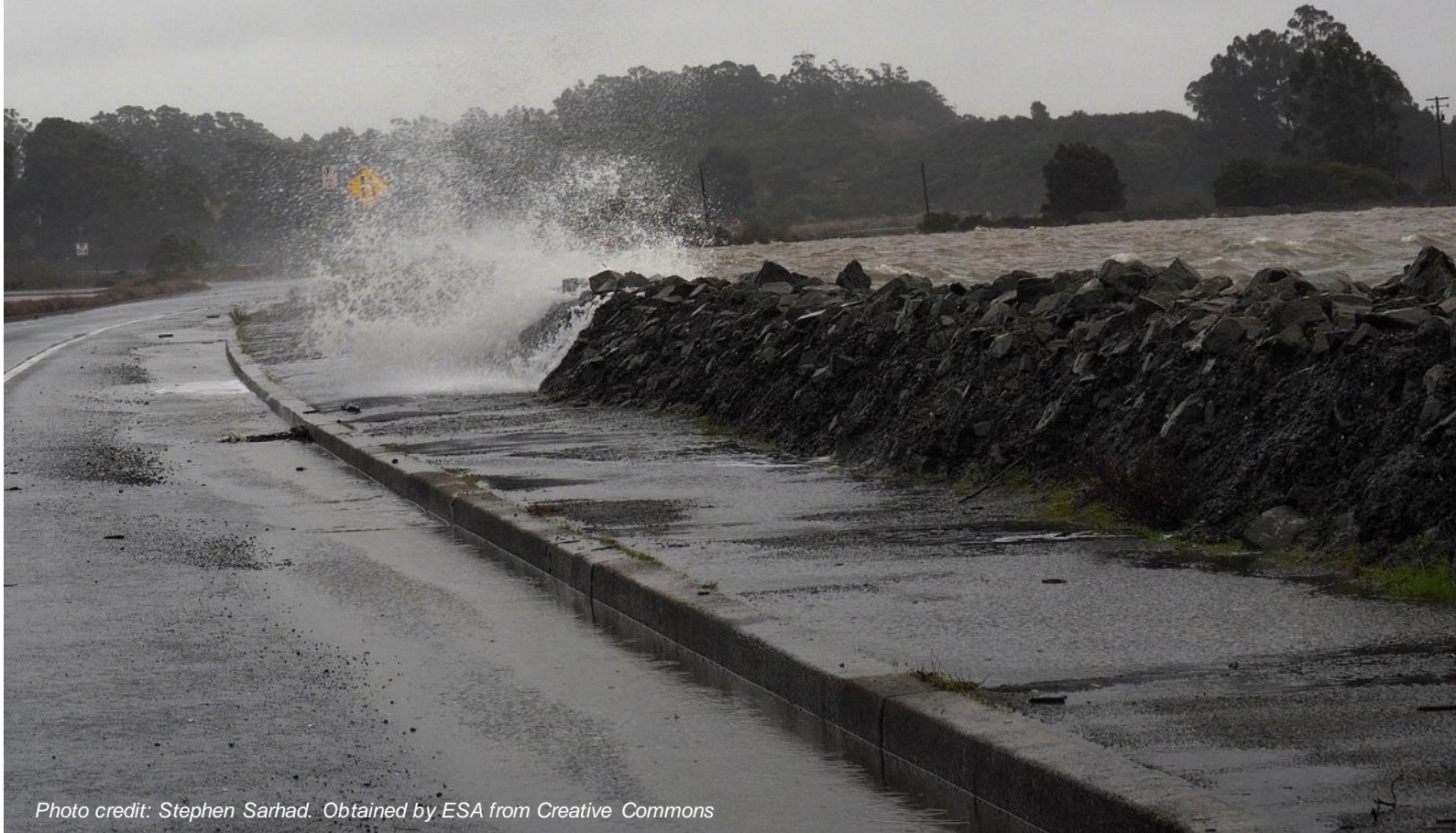
Figure A9 Flooding observed from combined high tides and wave runup at Pt San Pedro Road
