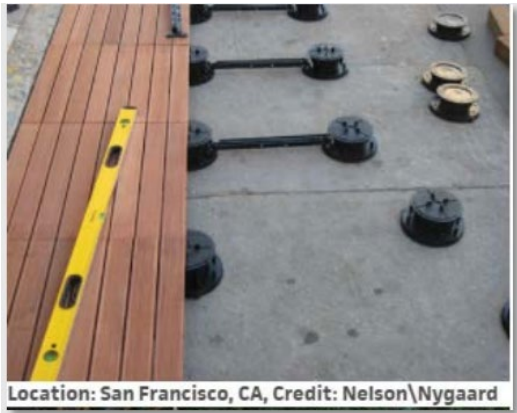
Figure 2: Bison pedestals for streetary sub-structure
