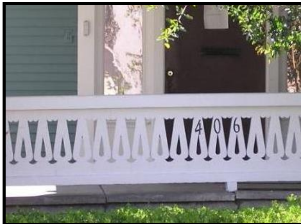
Colonial Revival Porch Detail
