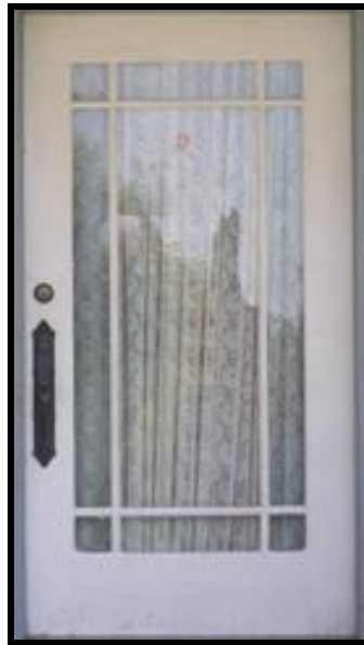
Colonial Revival Door
