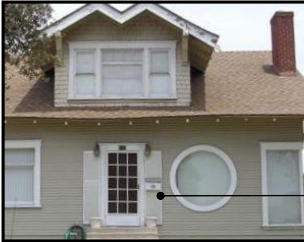
Enclosure of Front Porch and Installing Shutters at Front Door
