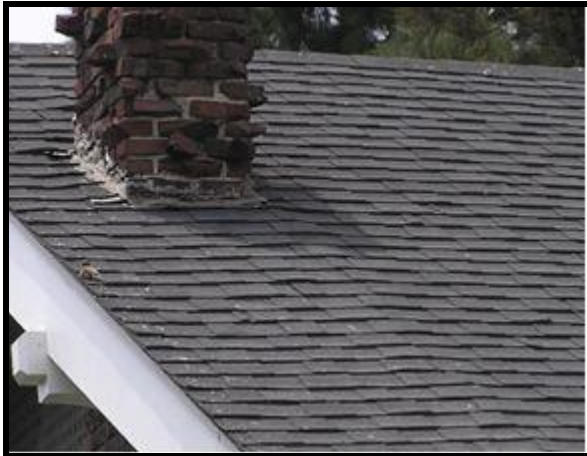
Asphalt Shingle Roof
