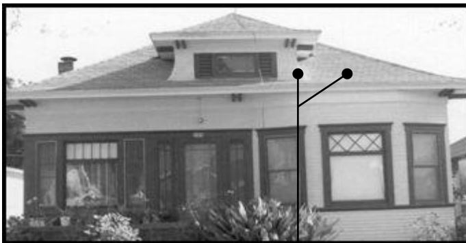
Hipped Roof with Dormer
