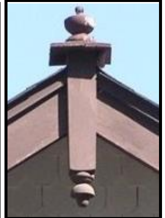
Bungalow Roof Detail
