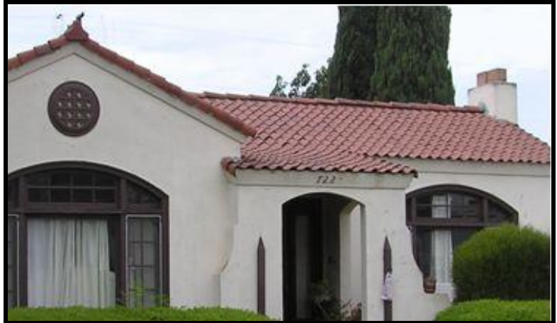
Spanish Tile Roof
