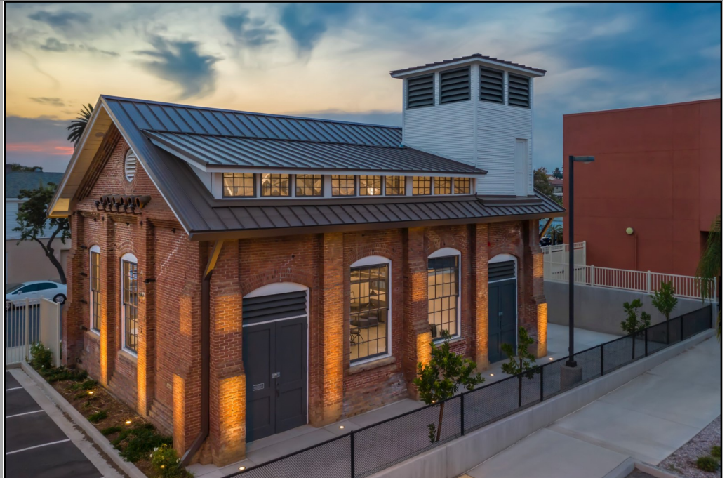
Imagen de arriba: Pacific Electric Sub-Station No. 14, 2020 Historic Preservation Award Winner (SAUSD)
