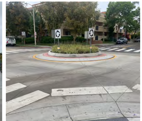
Existing traffic circle on 16th Street
