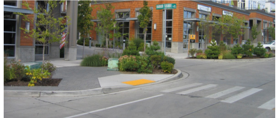
Bulb Out / Curb Extensions
