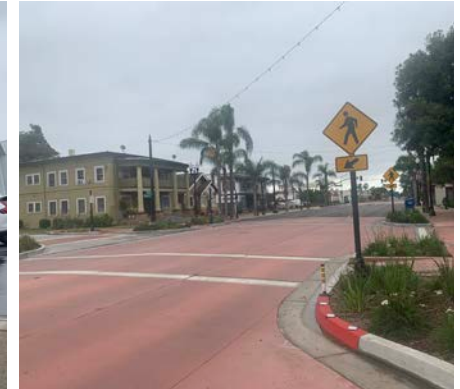
Curb extensions on Main Street
