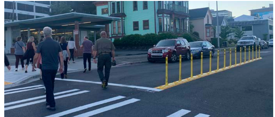
Hardened Centerlines with Flexposts
