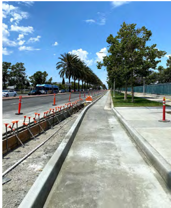
Bristol Street Protected Bike Lane
