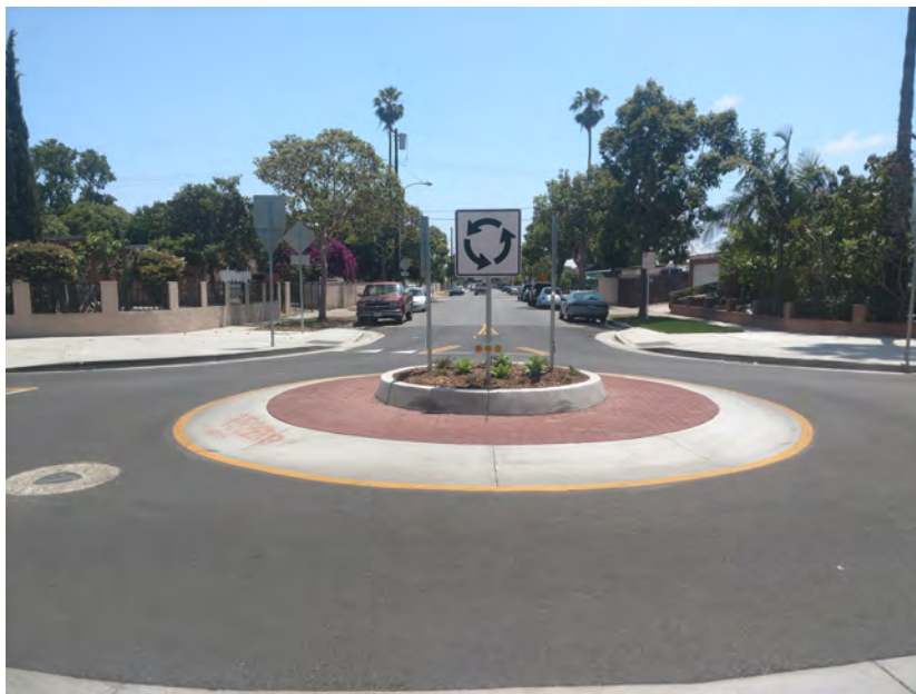
South Pacific Ave and West Willits St Roundabout
