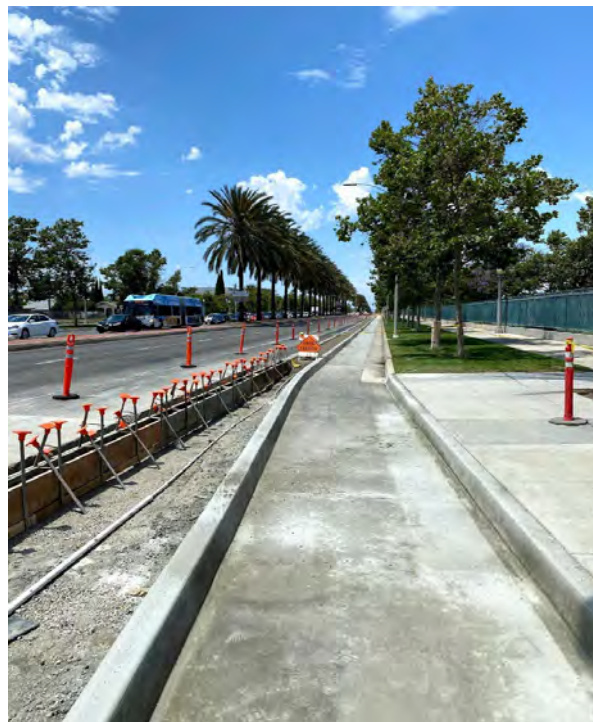
Bristol Street Protected Bike Lane
