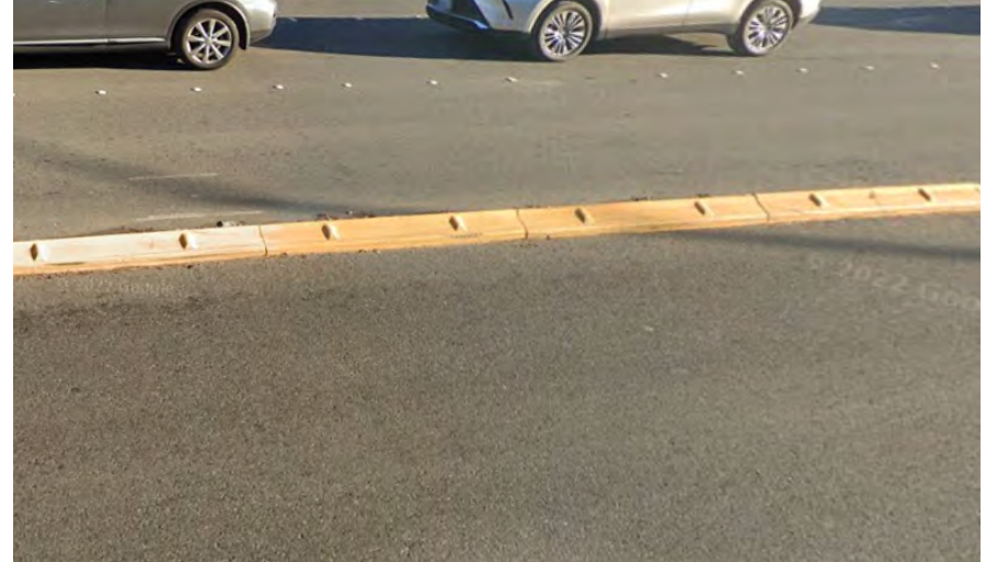
Type C Curb, sourced from Google Maps
