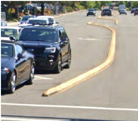
Type C-Curb used in the City of Bellevue, WA Source: Google Maps
