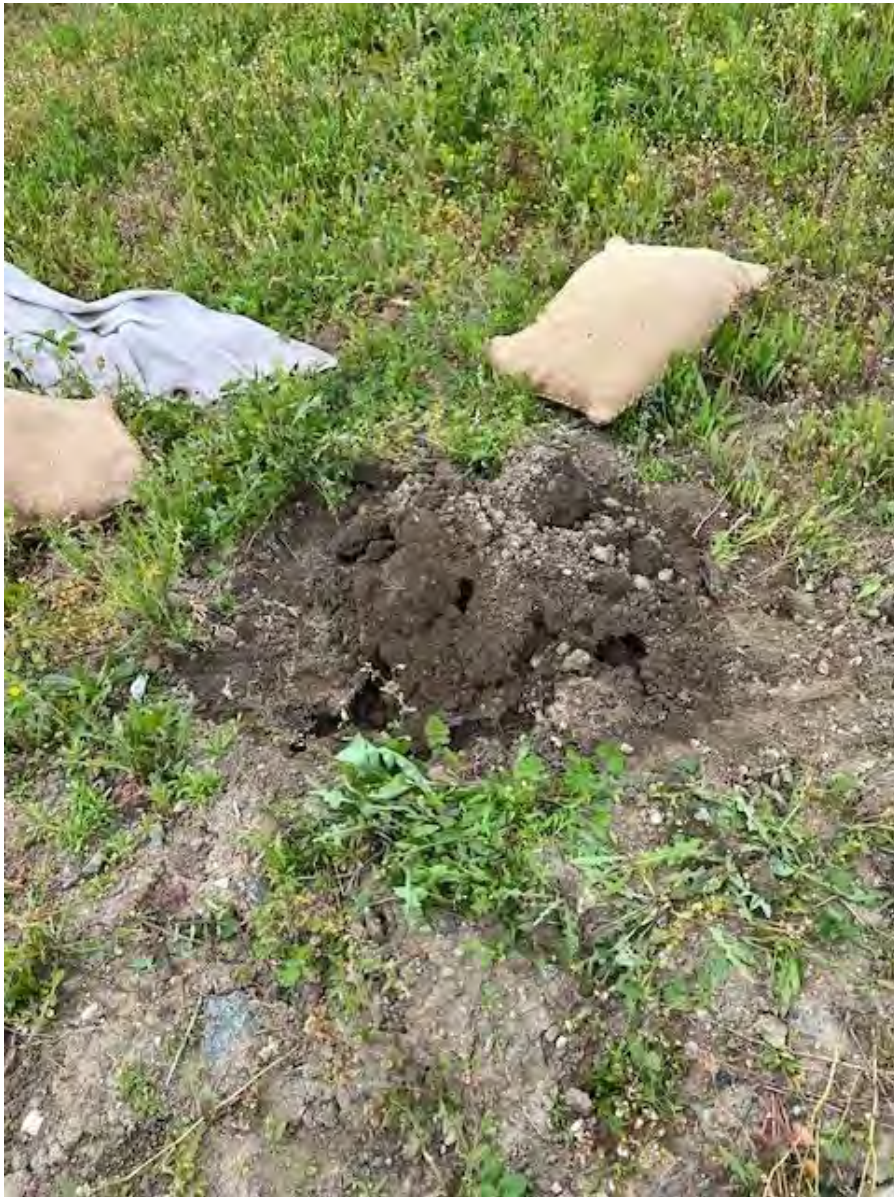
Soil Beneath Stray Vent Cap
