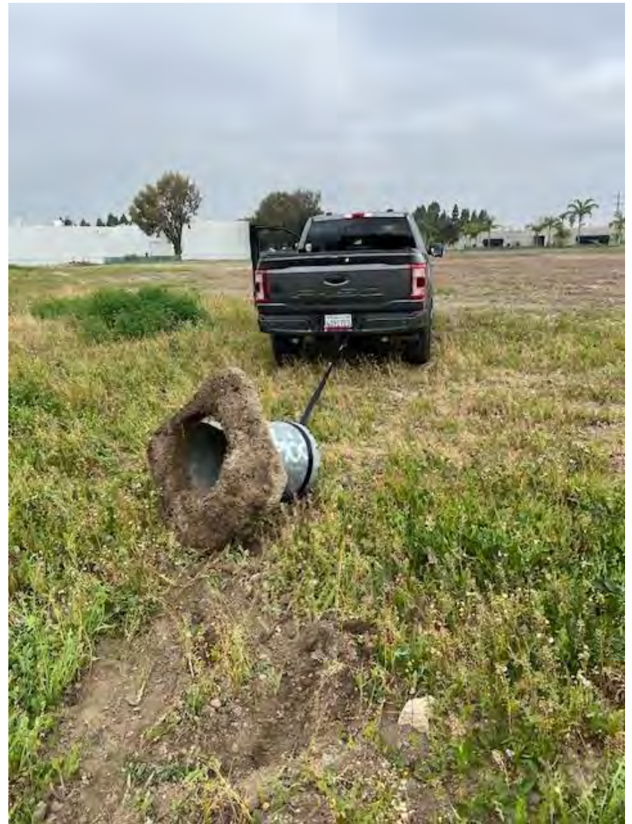
Stray Vent Cap Being Removed
