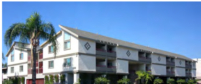
Ross Street Apartments
