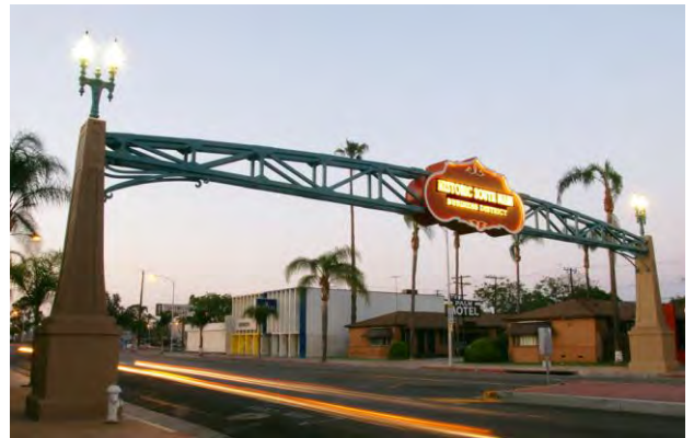
Historic South Main Business District Archway
