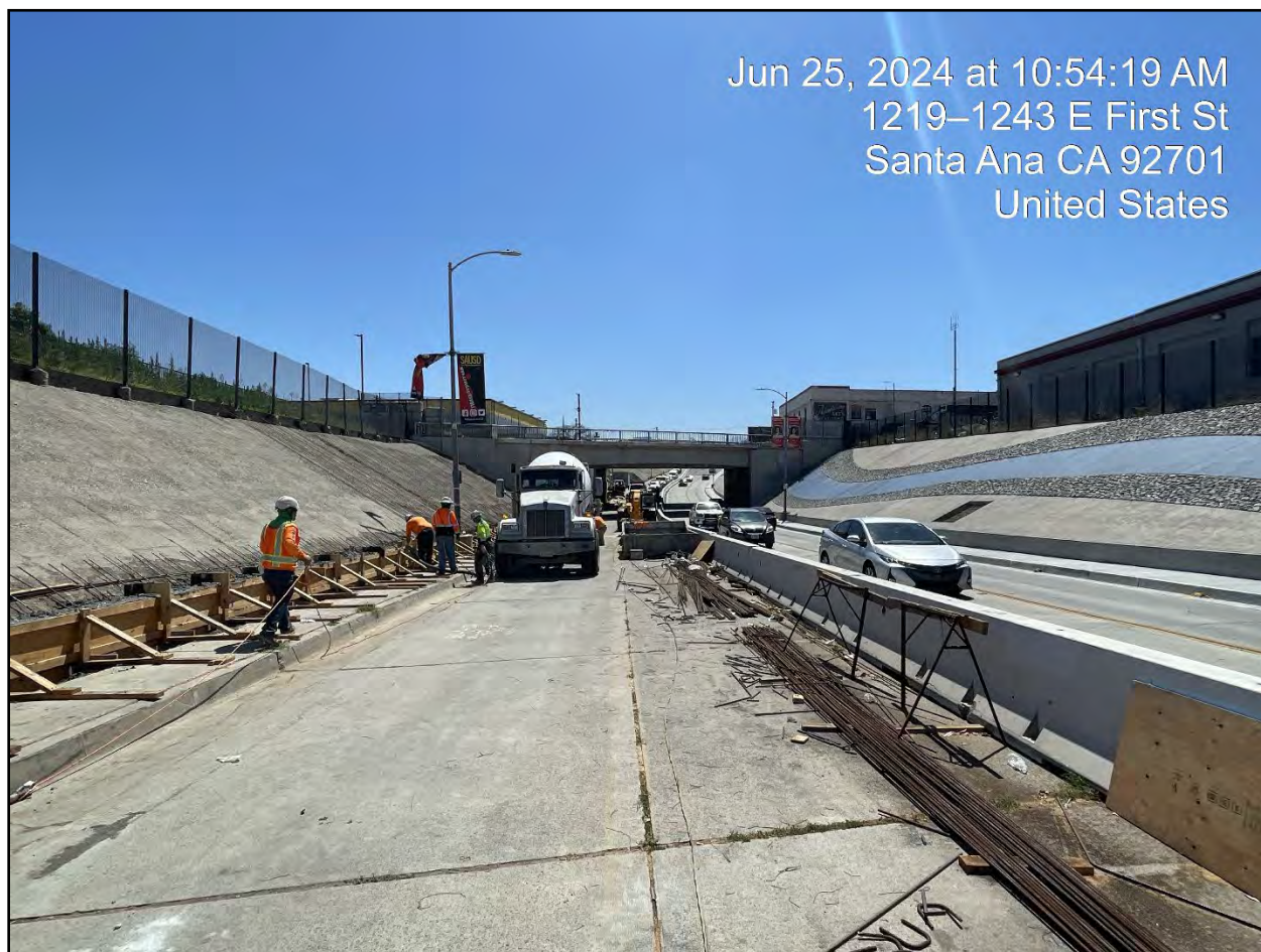
Photo 1: Installation of concrete anchor wall on northern slope. Southern slope substantially completed
