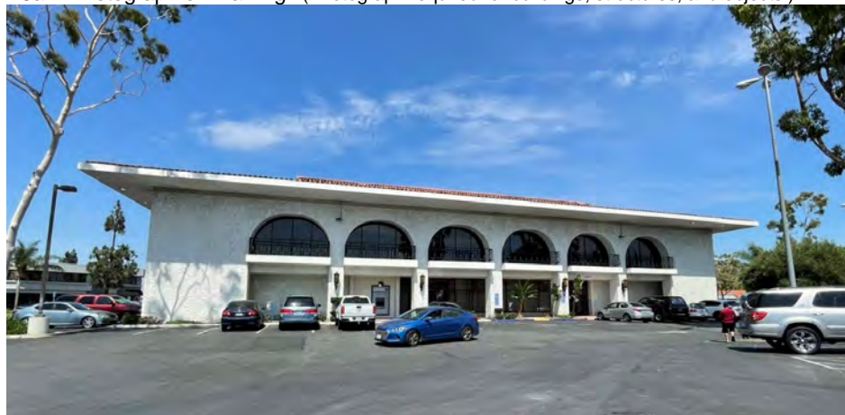
P5a. Photograph or Drawing (Photograph required for buildings, structures, and objects.)
