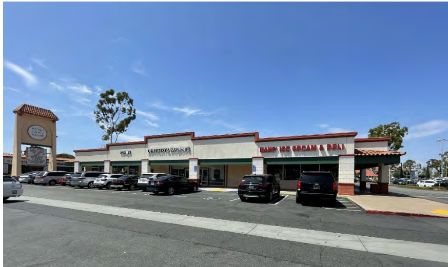
Aerial view of Building B
