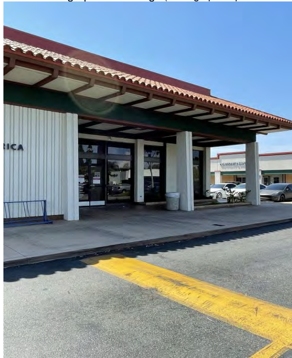
P5a. Photograph or Drawing (Photograph required for buildings, structures, and objects.)
