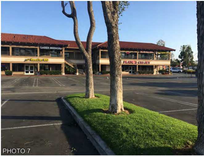
PHOTO 7 SOUTHERN PORTION OF PROPERTY, VIEW LOOKING NORTH WITH 3814 AND 3816 S BRISTOL ST IN BACKGROUND
