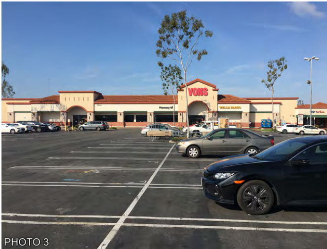
PHOTO 3 NORTHERN PORTION OF PROPERTY, VIEW LOOKING WEST AT VONS FROM EASTERN BOUNDARY
