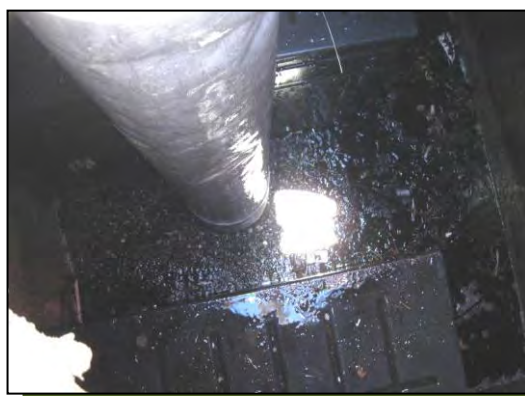
Removal of trash, sediment and debris.
