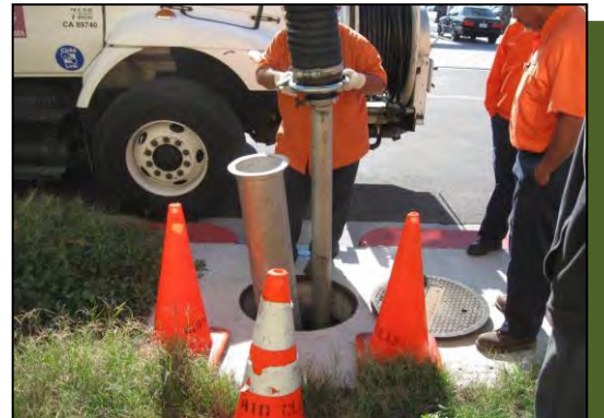
Insertion of vacuum hose into separation chamber.
