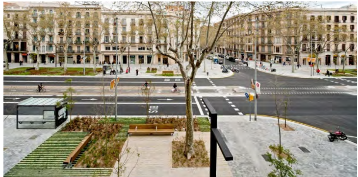
Imagery Source: Project Design Team
