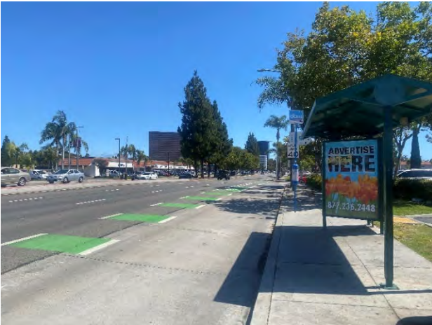
Bristol Street Existing Condition
