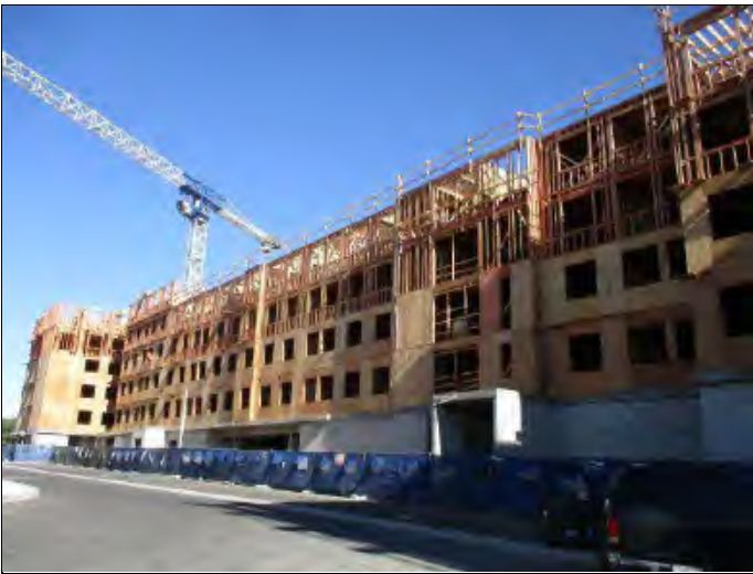
21. Adjacent property - east
