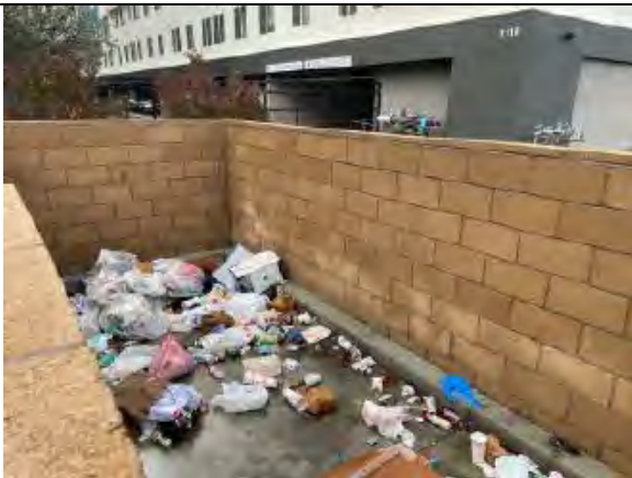
5. Consumer debris located within trash enclosure on eastern portion of Subject Property
