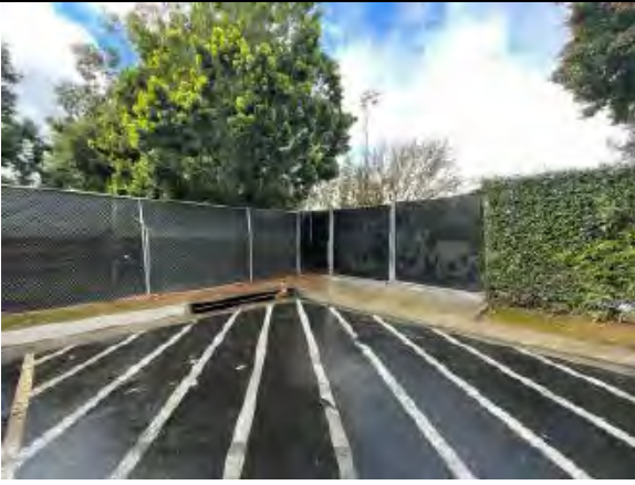
7. Gate leading to adjoining property near southwestern corner of Subject Property
