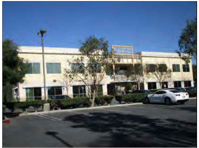
22. Adjacent property - west
