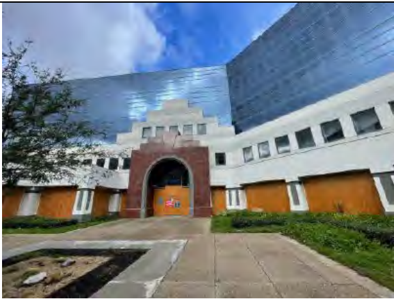
3. Boarded entrance located on eastern portion of Subject Property (2)
