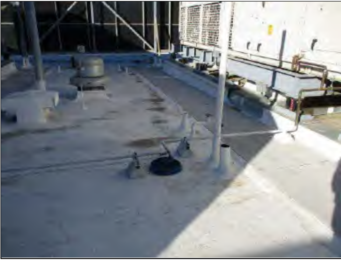
19. Typical roof drain
