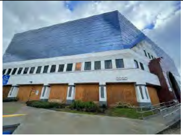
8. Boarded northern entrance to Subject Property
