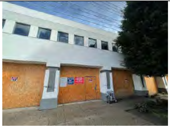
4. Boarded entrance located on southern portion of Subject Property
