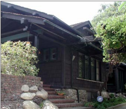
Combination stone and brick base
