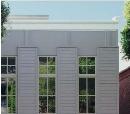
Parapet with cornice
