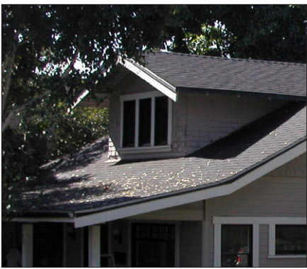
Dormer window with pitched roof
