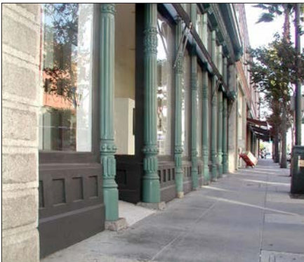
Storefront with cast iron columns
