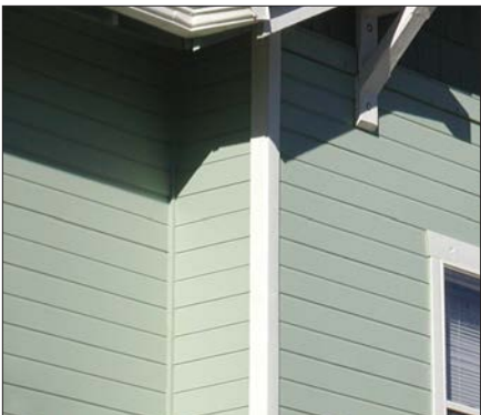
Painted horizontal wood siding
