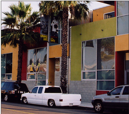
Concrete block base
