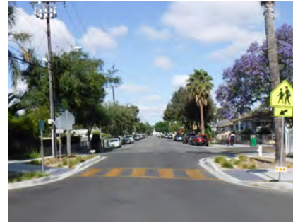
Pacific Electric Bicycle Trail Crossing Central Avenue
