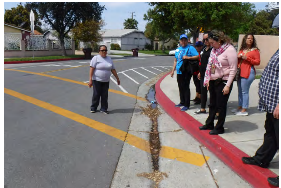
Without a curb ramp, crossings like this one by Sepulveda Elementary School present barriers for people using strollers, wheelchairs, or other mobility devices.
