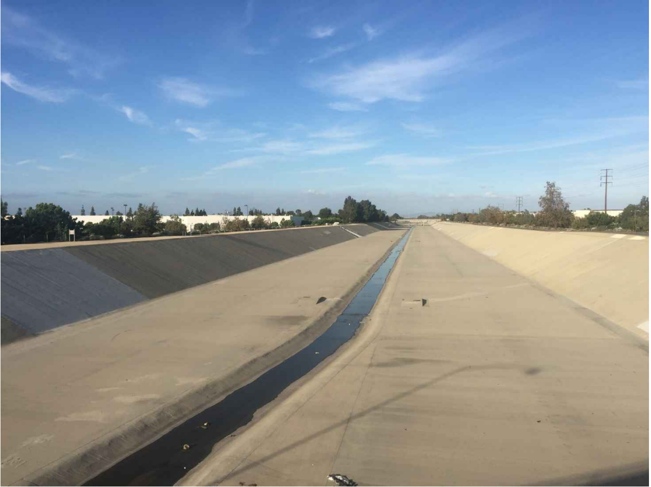
Figure 3-28: Santa Ana River View upstream from Talbert Avenue Bridge in Fountain Valley. The portion of the river here has both concrete levees and bottom.
