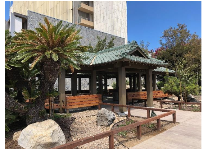
Civic Center Improvements: Pavilion Renovation
