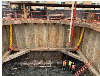
San Lorenzo Sewer Lift Station
