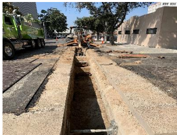
Bush Street Water Main Improvements
