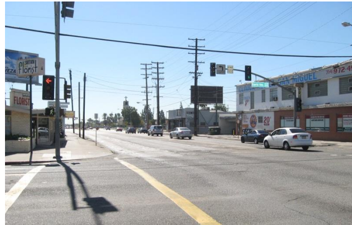
Intersection of Bristol Street and Santa Ana Boulevard looking south, before street widening, November 2010.
