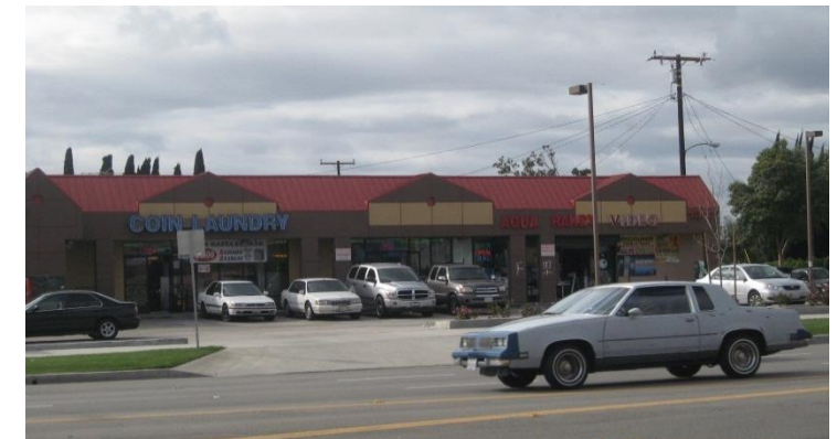
Commercial center on Bristol Street and Third Street, after completion of street widening, February 2011.
