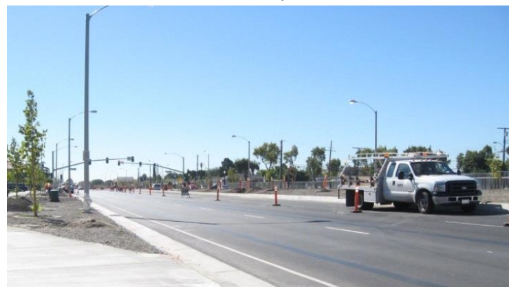
Construction on Bristol Street during street widening project in, November 2010.
