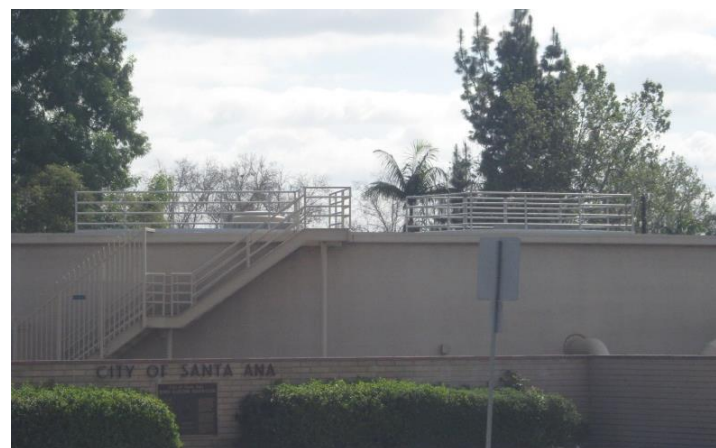
The city owned water reservoir on Bristol Street near Seventeenth Street, February, 2011.
