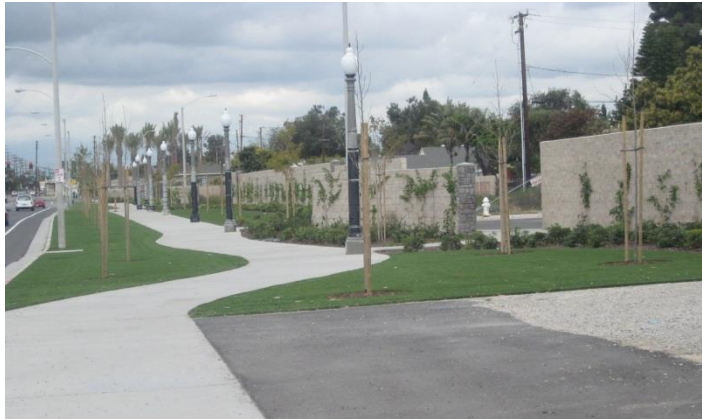
Completed portion of Bristol Street, February, 2011.
