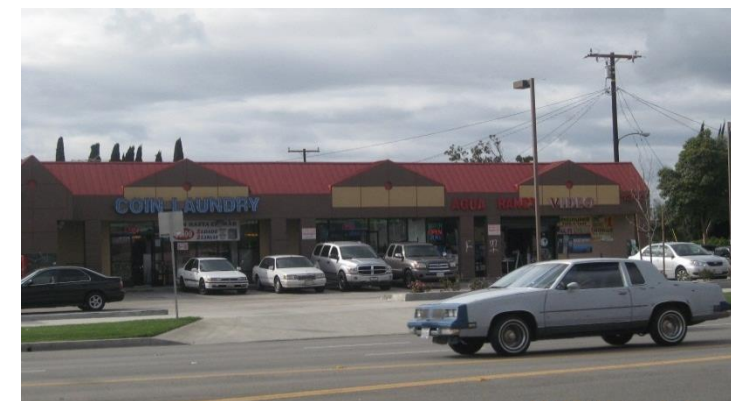
Commercial center on Bristol Street and Third Street, after completion of street widening, February 2011.
