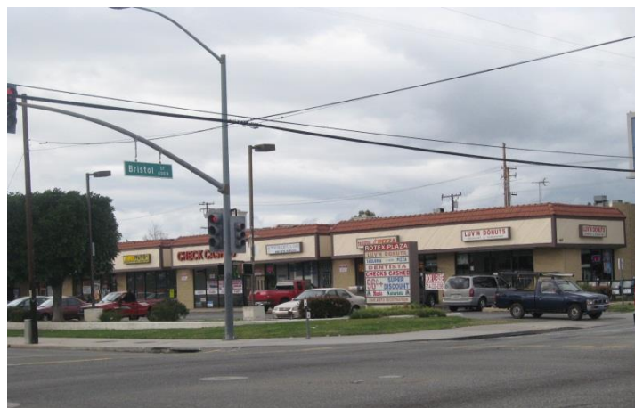
Commercial center on Bristol Street and Santa Ana Blvd before street widening, February 2011
