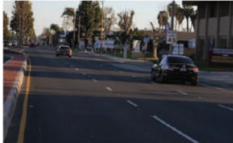
N Fairview Street experiences high vehicular speeds
