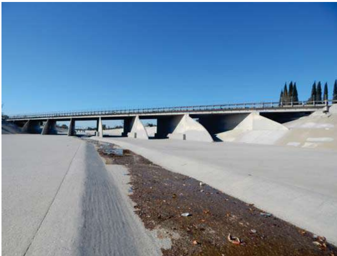
View of concave low flow channel in center of the channel bed with standing water.
