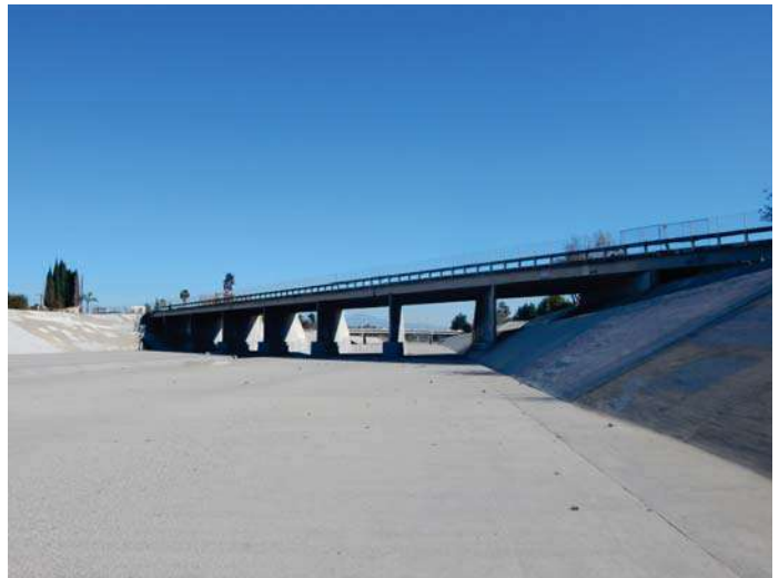
View of channel bed and bank, looking southeast.
