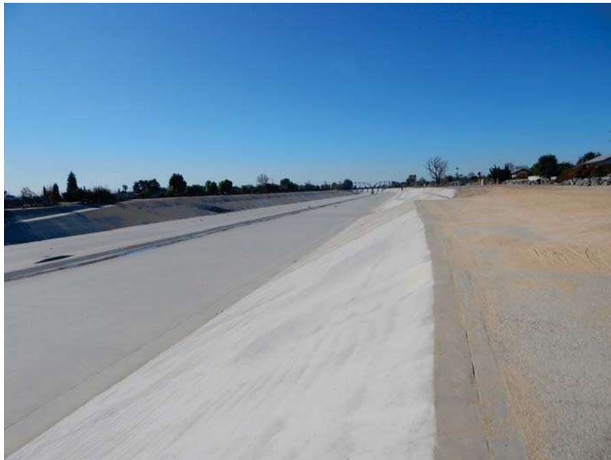
View downstream of the existing Fairview Street Bridge, showing the proposed construction access route on the north side of the Santa Ana River.
