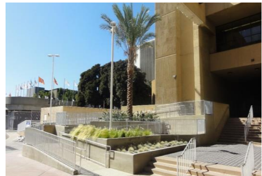
Civic Center ADA Access Ramp
