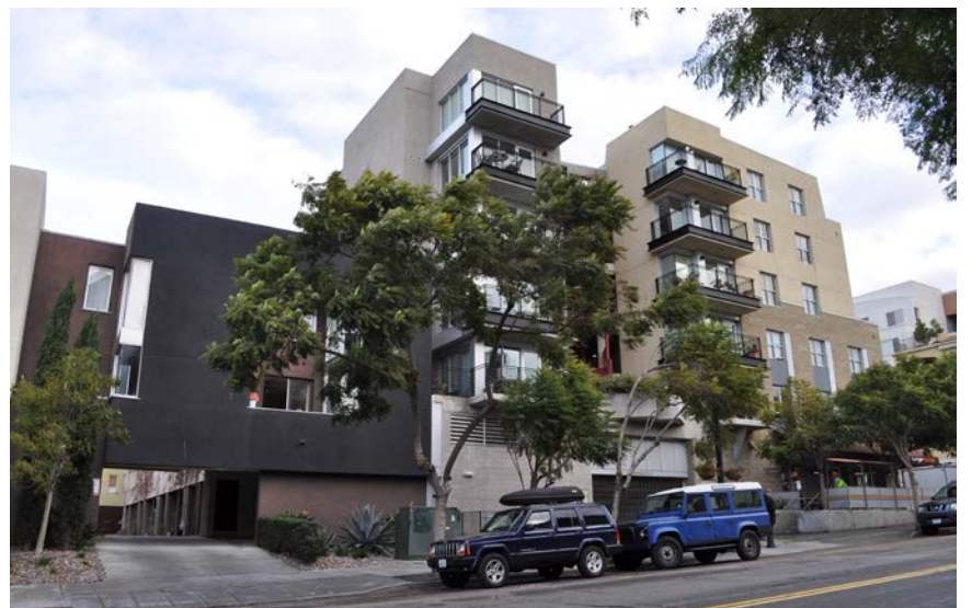
Parking lots and structures should be screened and designed so that they enhance the pedestrian environment. Garage openings should adhere to the overall aesthetic of the building's architecture.
