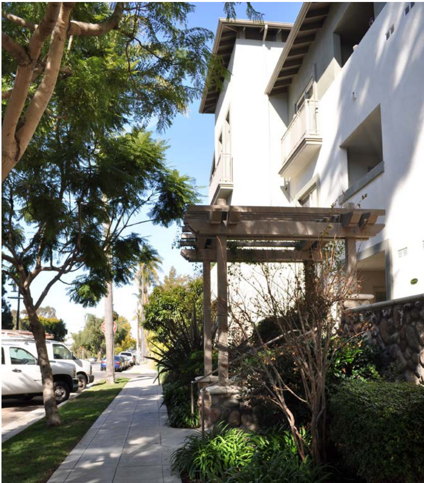
Trees and landscaping should be used to enhance the pedestrian environment and buffer the setback.
