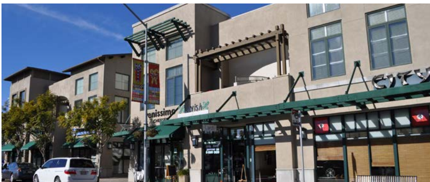
Awnings provide visual interest for the pedestrian and automobile while also providing shade for the frontage and sidewalk.
