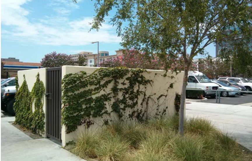
Trash and recycling enclosures should use the same materials as the primary building and screen the area employing elements such as solid masonry walls, berms, and landscaping.
