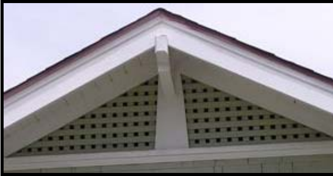
Bungalow Attic Vent
