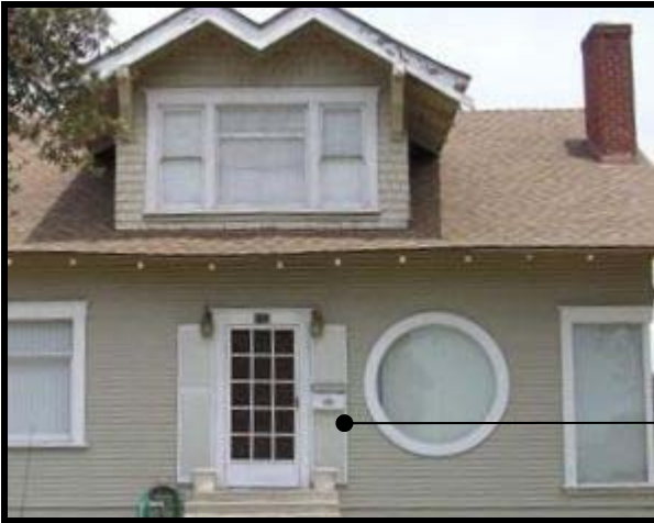
Enclosure of Front Porch and Installing Shutters at Front Door
