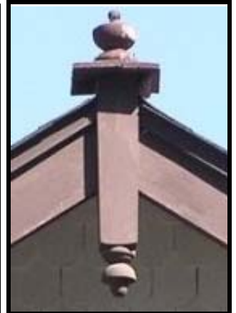
Bungalow Roof Detail
