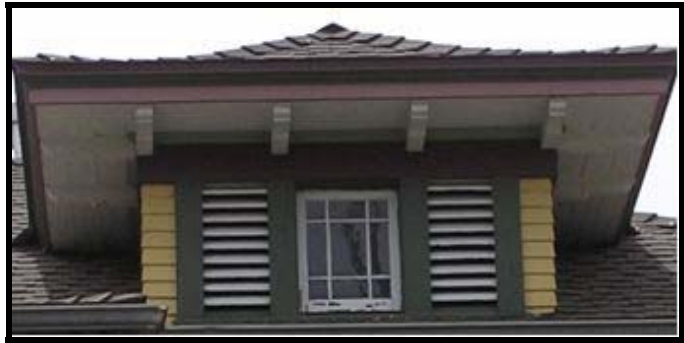
Colonial Revival Attic Vent
