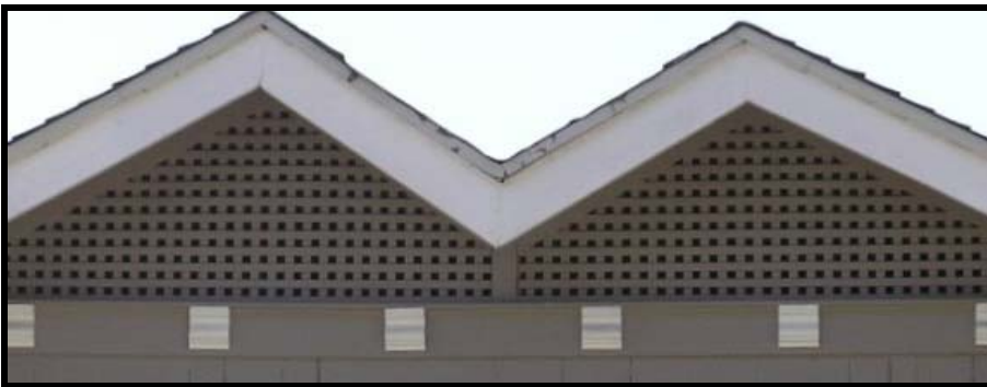
Craftsman Bungalow Attic Vent
