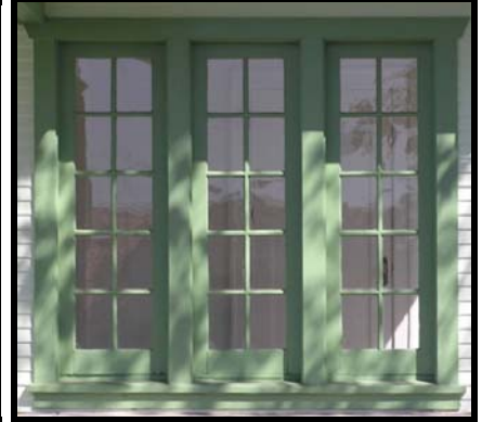
Casement Windows with Lights
