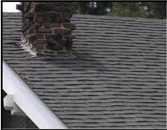
Asphalt Shingle Roof
