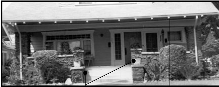
Brick and Stone Porch
