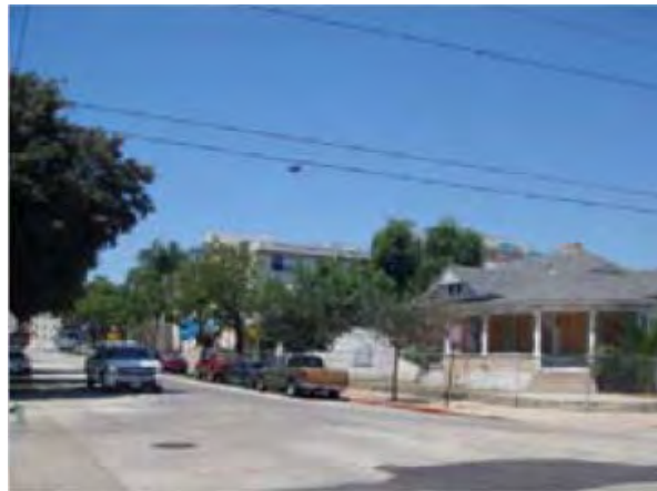
20. View of boarded up single-family residence on corner of Mortimer Street and 5 th Street (Area F).
