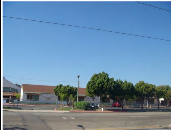
11. View of Carver Elementary School looking north from across Santa Ana Boulevard.
