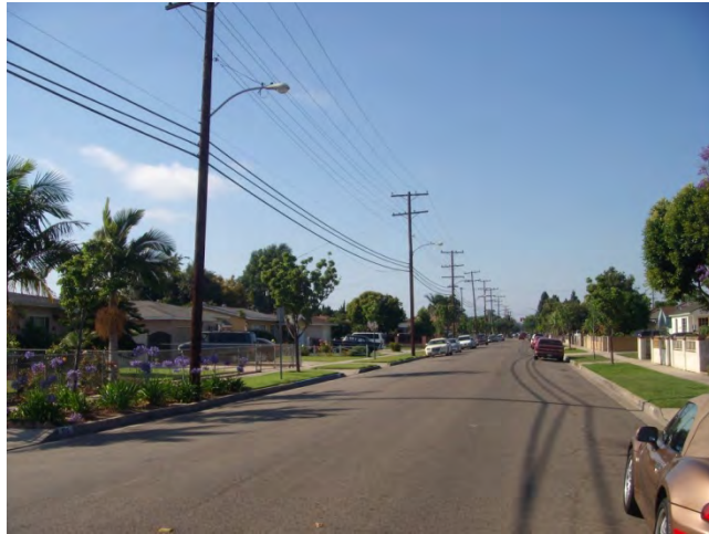
7. Residential neighborhood adjacent to industrial facilities, looking north on English Street from 5 th Street.
