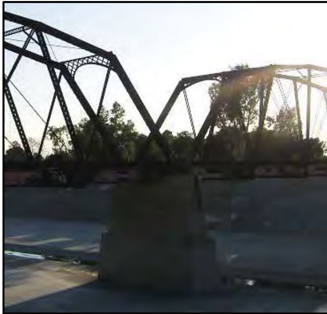
Detail of riverbed pier and cross-bracing. View looking Southwest.
