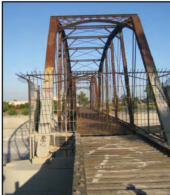
Detail of west portal highlighting the through style. View looking East.
