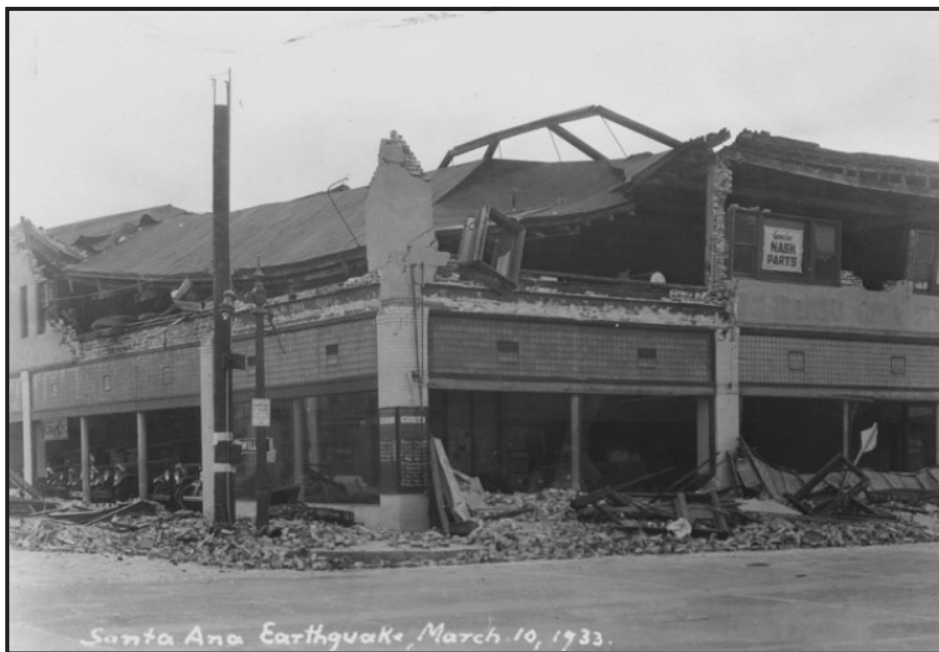
Earthquake damage on the corner of Fifth and Bush Streets Santa Ana, March 10, 1933 [Santa Ana Public Library]
