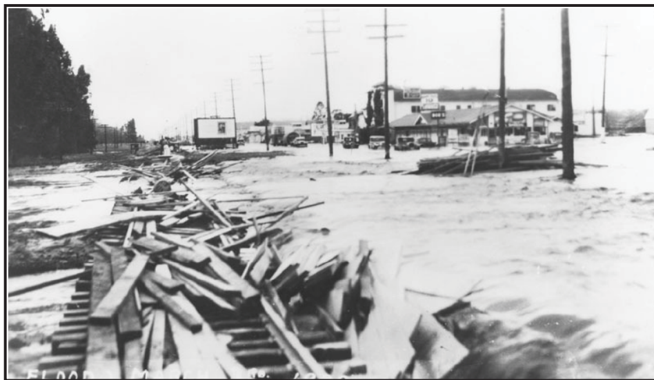
Railroad track damage, Santa Ana River flood, Orange, California, March 3, 1938 [Orange Public Library]
