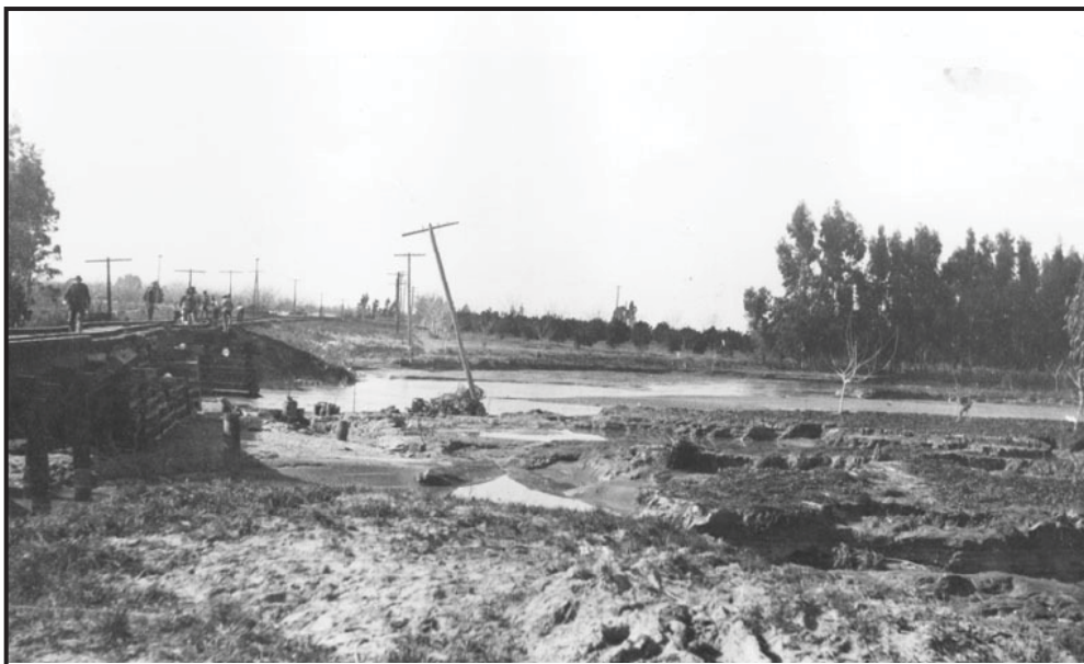
Flood damage to Santa Fe Railroad tracks and bridge, Orange, California, 1916 [Orange Public Library]
