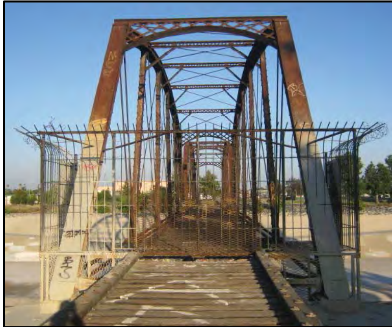
Detail of west portal, deck, and truss. View looking East.
