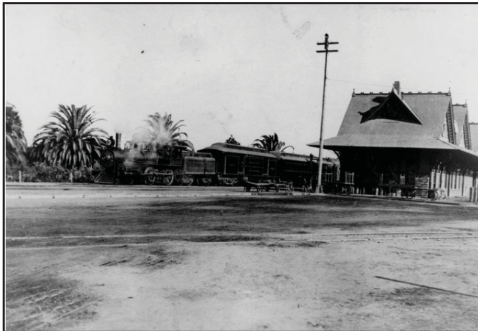
Santa Fe Railway Depot, Santa Ana, c. 1905 [Santa Ana Public Library]
