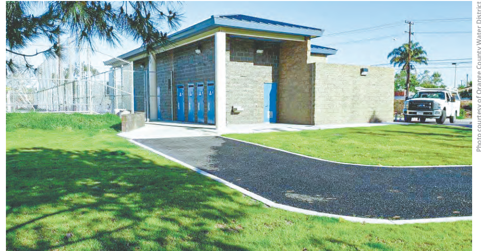
Photo courtesy of Orange County Water District
