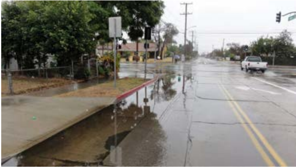
Civic Center Dr and Raitt St – December 22, 2016 Storm
