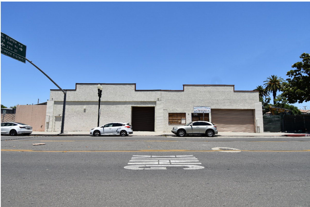
Figure 3.1-8 Southern View of Block B from 4 th Street
