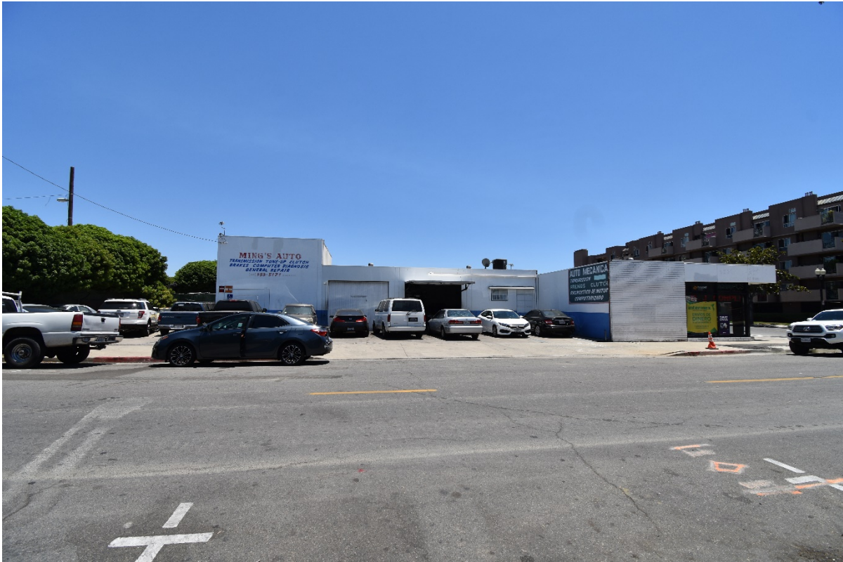
Figure 3.1-7 Southwest View of Block B from 4 th Street and Mortimer Street
