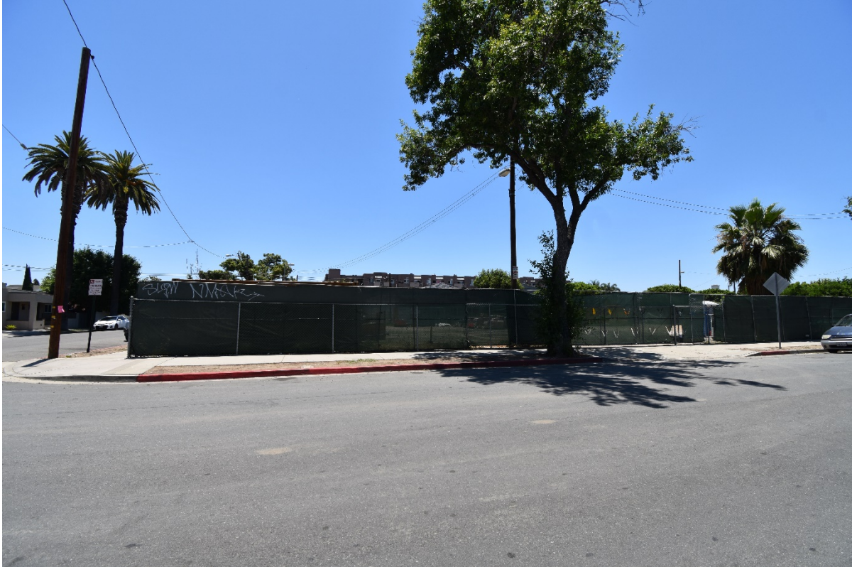
Figure 3.1-5 Northeastern View of Block B from 5 th Street and Minter Street
