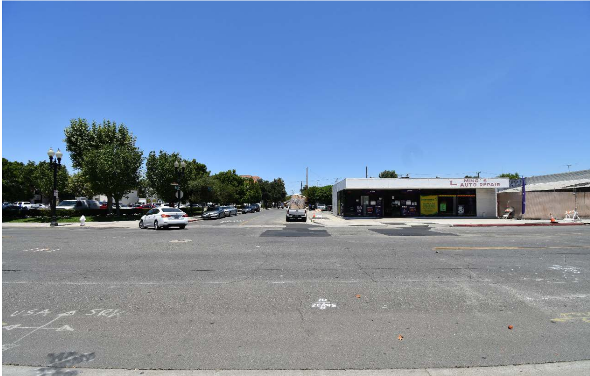
Figure 3.1- 3 Southern View of Blocks A and B from 4 th Street and Minter Street
