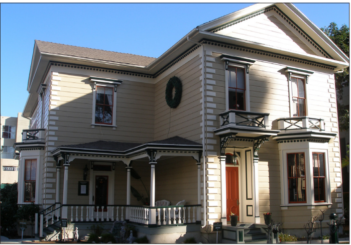
Illustrative Photo: Duplex with Porch Frontage
