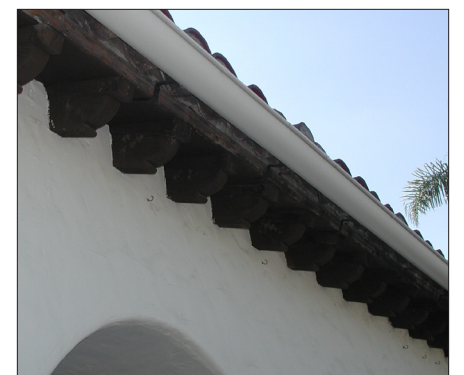
Rustic wood cornice
