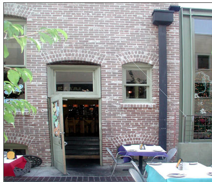
Downspout on back side of building;
