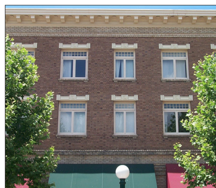
Grouped second-floor windows
