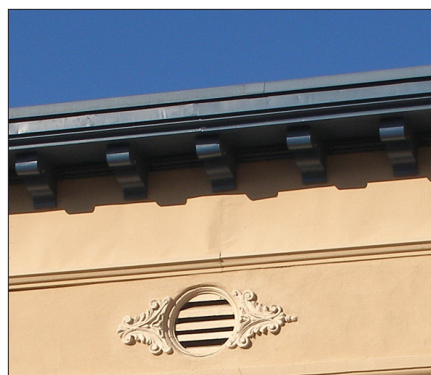
Parapet and wood cornice
