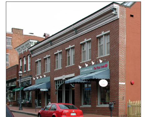
Drainage imbedded in exterior wall
