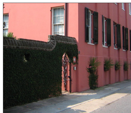
Integral 1-story wall with doorway
