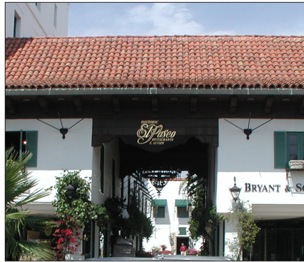
Sloped tile roof
