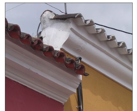
Tile on profiled parapet
