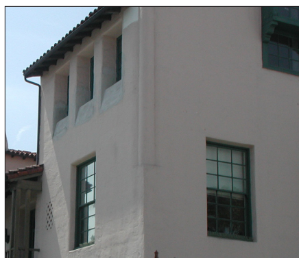
Deep, recessed openings
