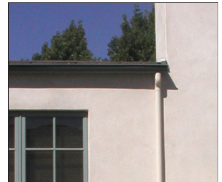
Gutter and downspout
