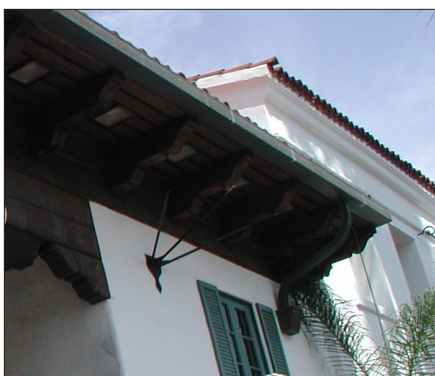
Expressed rafters, broad eave
