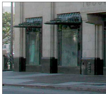
Masonry base and monolithic wall
