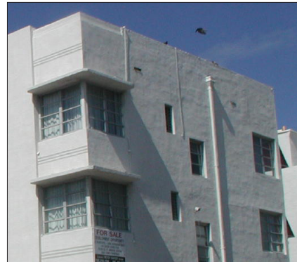
Scupper and downspout on building side
