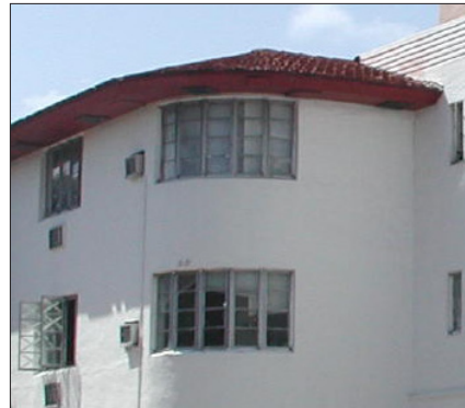
Sloped roofs without gutters
