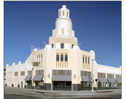
Corner stepped tower
