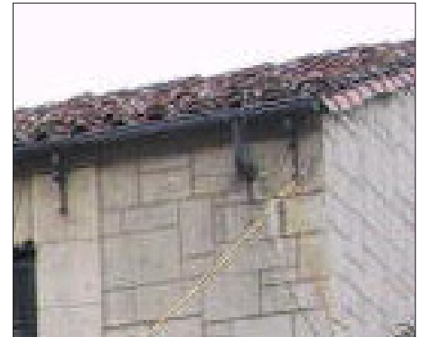
Gutter with downspout into wall
