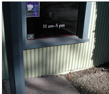
Corrugated siding to grade
