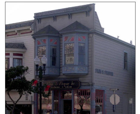
Projecting bay windows
