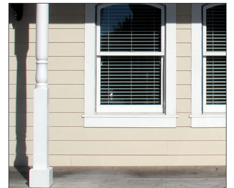
Wood plank siding to grade
