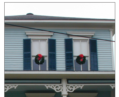
Double-hung windows on second floor
