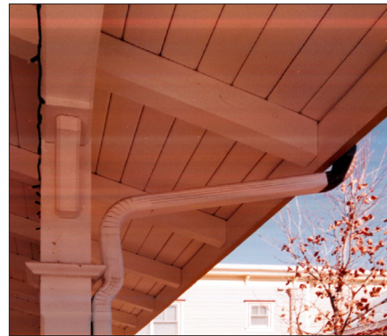
Gutter and downspout
