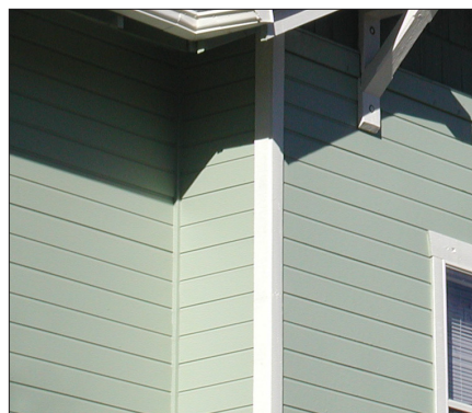
Painted horizontal wood siding
