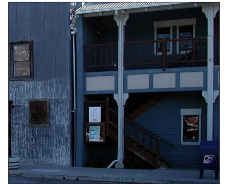
Gutter and downspout along column
