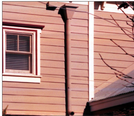
Scupper with downspout
