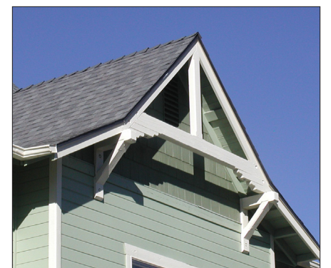
Gable with attic vents and combination of shingle and horizontal siding
