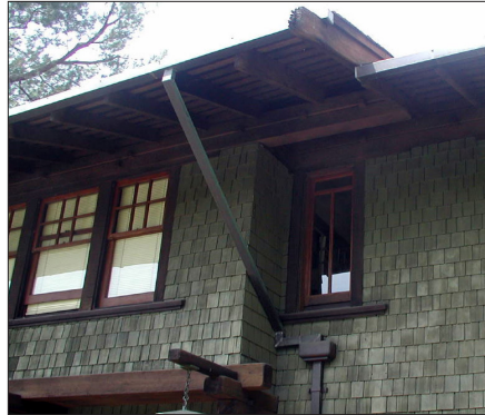
Gutter and downspout
