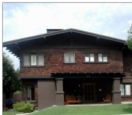
Unpainted siding above painted plaster
