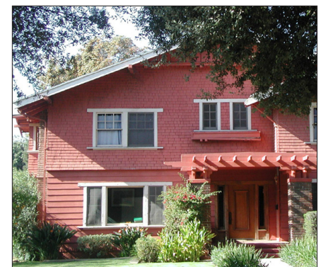
Painted shingles above painted lap siding
