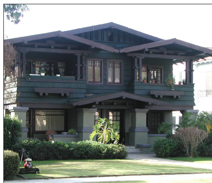
Siding above painted plaster
