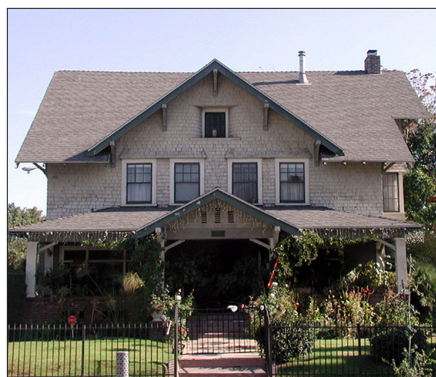
Intersecting gables with porch
