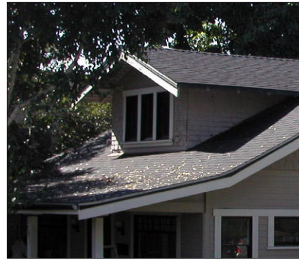
Dormer window with pitched roof
