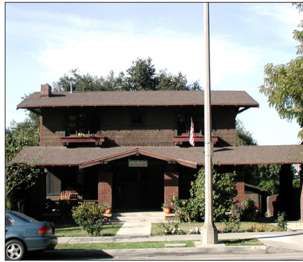
Roofs parallel to street
