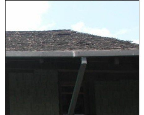
Gutter and downspout
