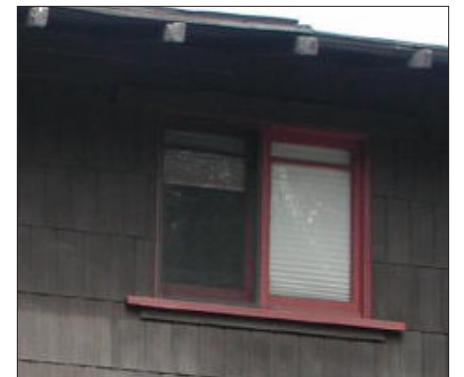
Paired openings composed horizontally
