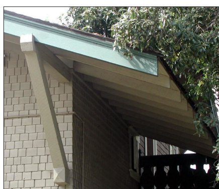
Brace and exposed rafters
