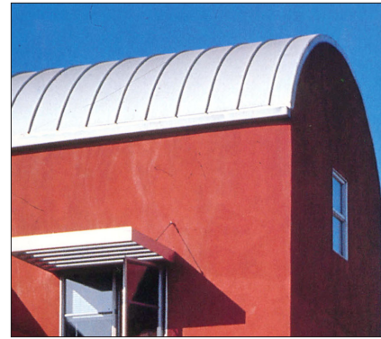
Metal barrel roof
