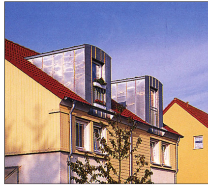
Sloped metal roof
