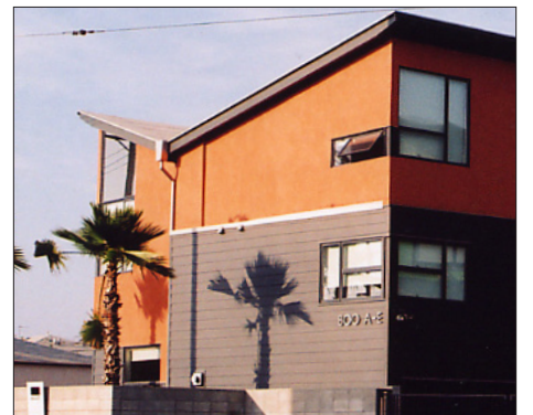
Plaster combined with siding
