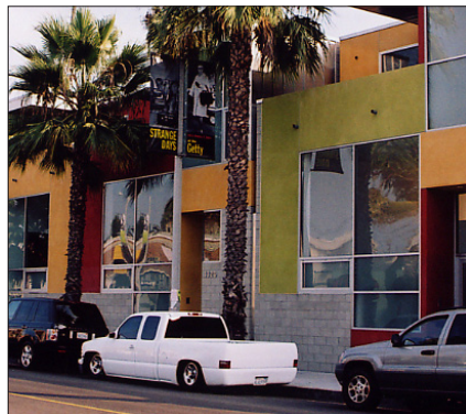
Concrete block base
