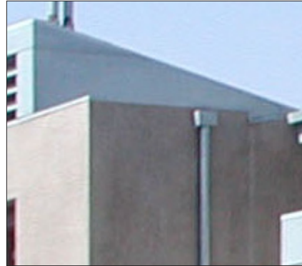
Scupper and downspout
