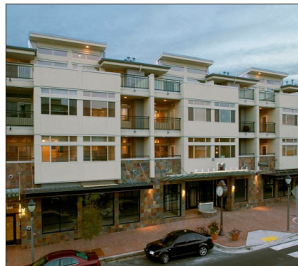
Ground floor as concrete base
