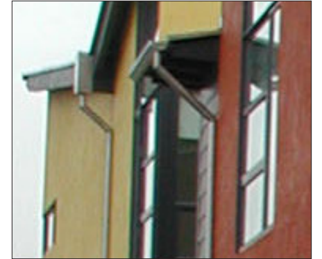
Scuppers and downspouts
