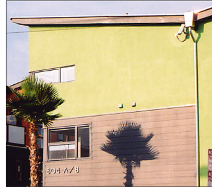
Scupper and downspout
