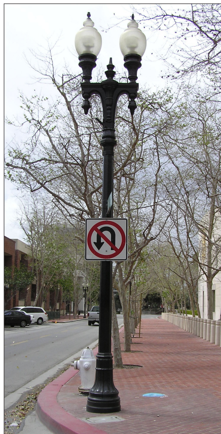
City of Santa Ana Standard Plan 1126 'A' 18' - 0" height to center of lamp refer to City specifications for details
