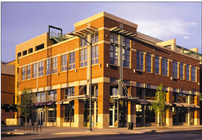
Illustrative Photo: Lined block with shopfront frontage
