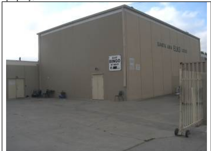
6. View of northwest corner of the subject property building.
