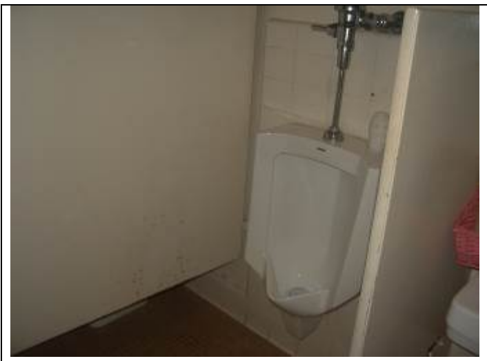
15. View of interior of a restroom at the subject property.
