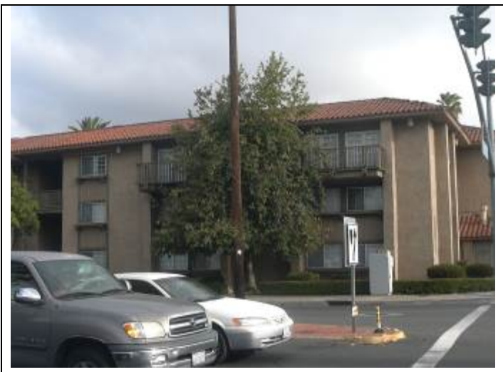
21. View of Saddleback Lodge north across 1 st Street.
