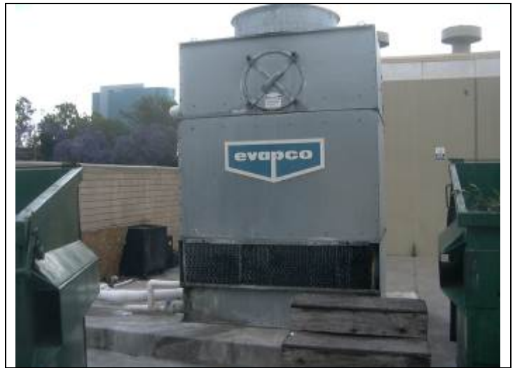
8. View of a cooling tower at the subject property.
