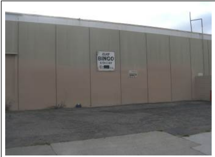
9. View of west side of the subject property building.
