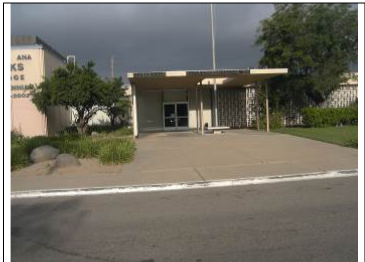
2. View of main entrance to the subject property building, east side.
