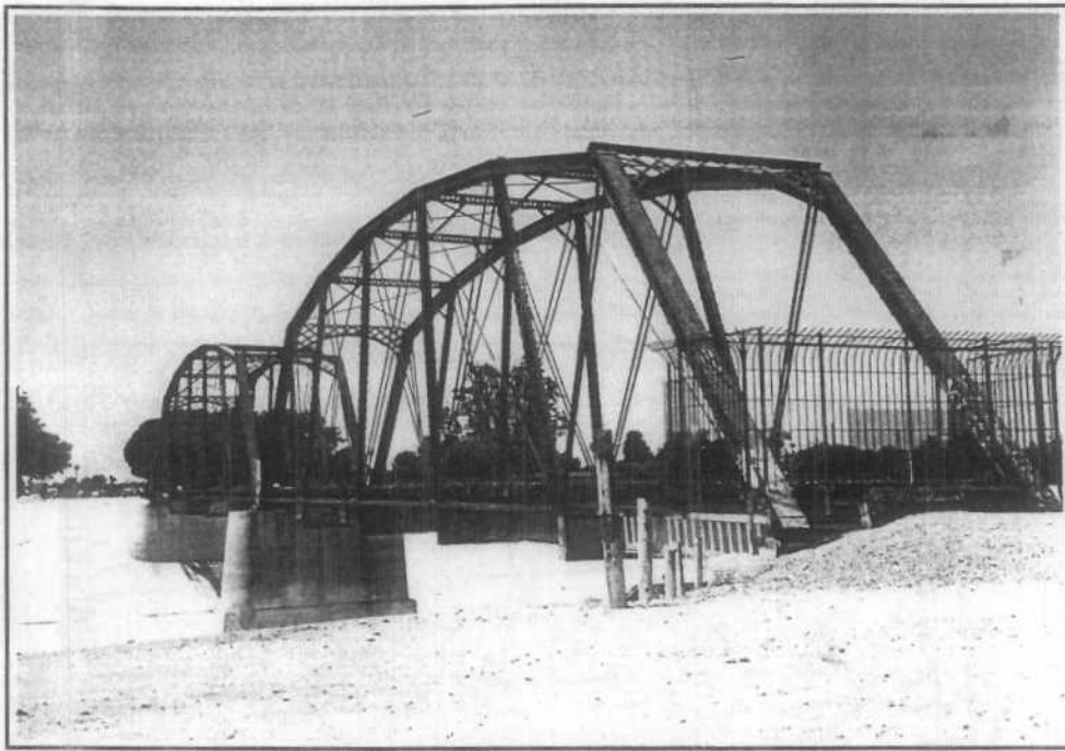
Pacific Electric Railway bridge over the Santa Ana River, looking northwest.
