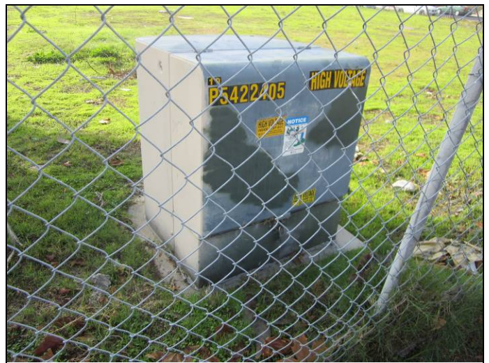
18. Transformer on subject property.
