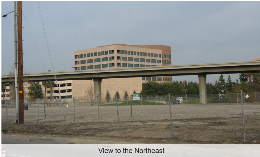
View to the North
