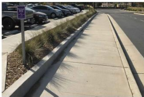
P1 CONCRETE PAVING TYPE 1 COLOR: NATURAL GRAY FINISH: MEDIUM BROOM JOINTS: TOOLED
